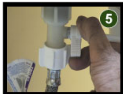
5 Fully insert the hose in the T-adaptor & tighten the nut with the tool (provided).
